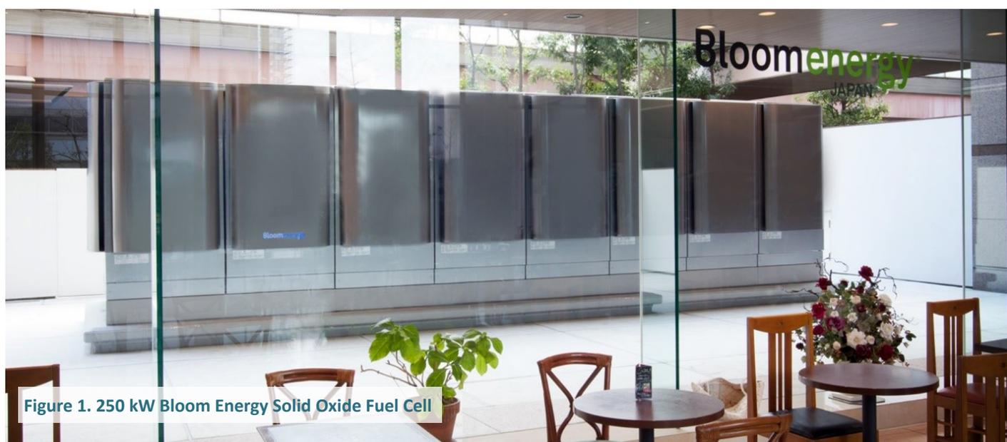
Figure 1. 250 kW Bloom Energy Solid Oxide Fuel Cell
