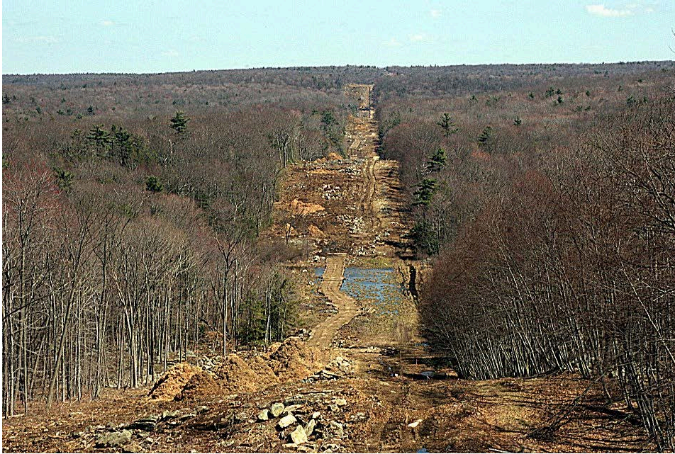
Swath cut through wetlands in Wawayanda State Park in northern New Jersey during the “300 Line Project” pipeline built by Kinder Morgan/ Tennessee Gas Pipeline Co.
