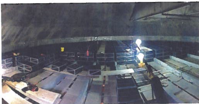
GORE® Mercury Control Modules being installed in a 500 MW scrubber.
