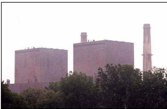
The Bowline plant in West Haverstraw.
