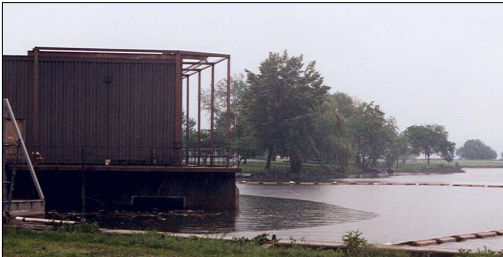
The cooling water intake structure at Bowline.
