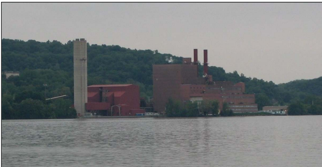
The Danskammer Plant in Newburgh, housing two old oil- and gas-fired units and two newer coal-fired units.
