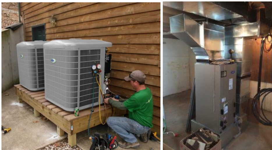
Figure 4. Ducted ASHPs collect heat with an outdoor unit and then use ducts to transport heat around the building.
