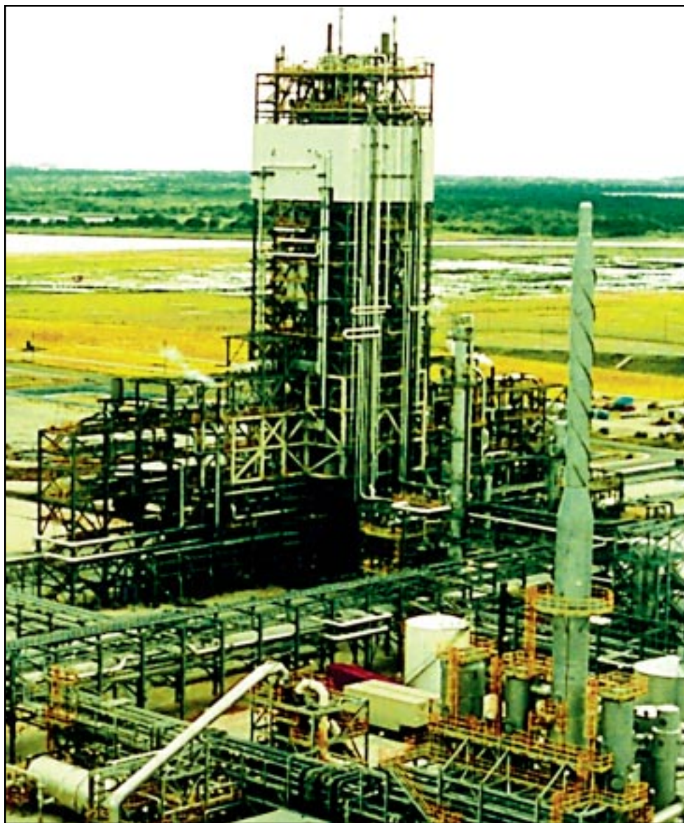
The sulfuric acid plant is located in the foreground and the gasifier and radiant syngas cooler are in the tall midground structure
