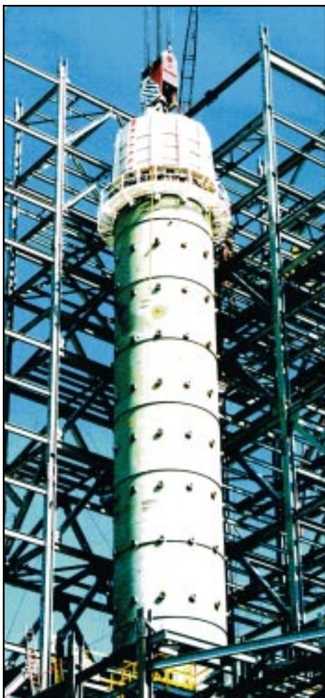
Installation of radiant syngas cooler
