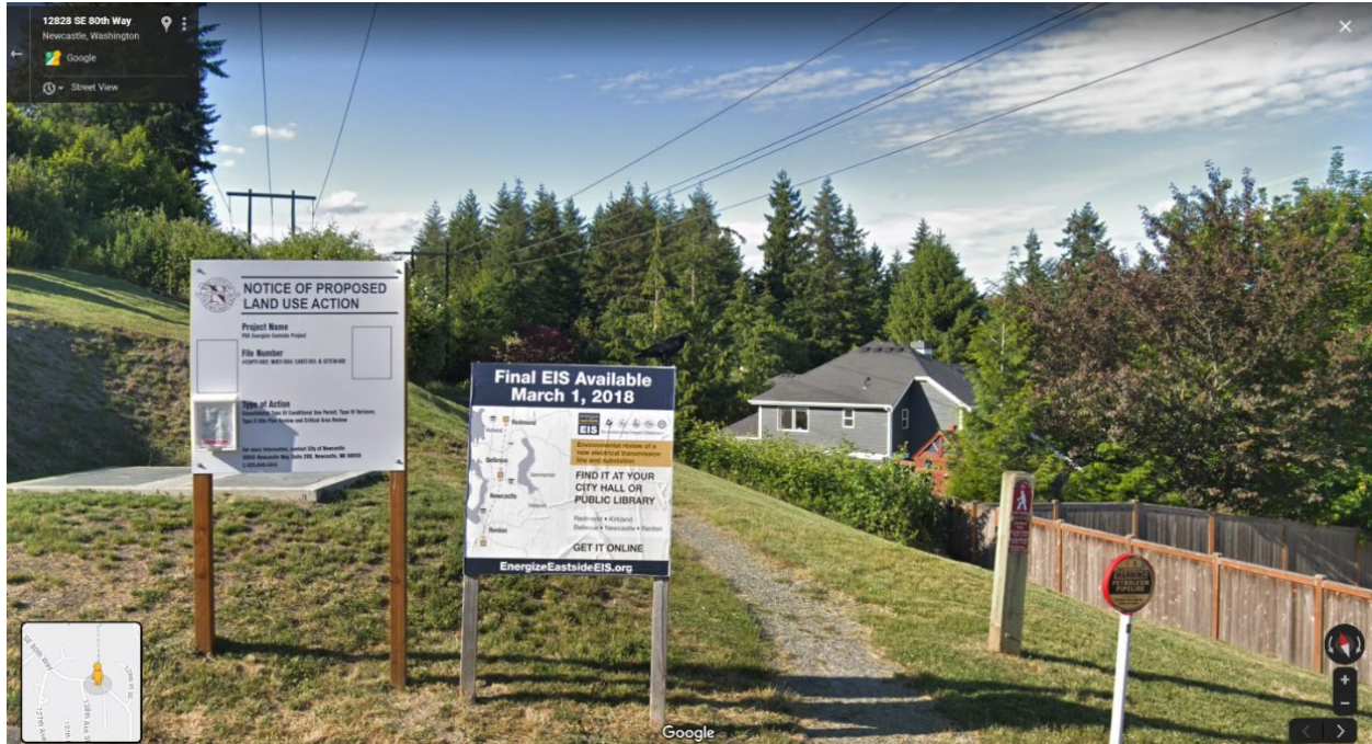
Figure 11. Existing two 115kV electric transmission facilities on H-frame poles travel in existing transmission corridor through Newcastle around SE 80th Way, Newcastle, WA 98056
