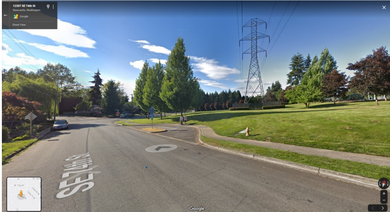
Figure 13. Seattle City Light 230kV Transmission Line at Donegal Park [SE 74th ST, Newcastle, WA 98056]
