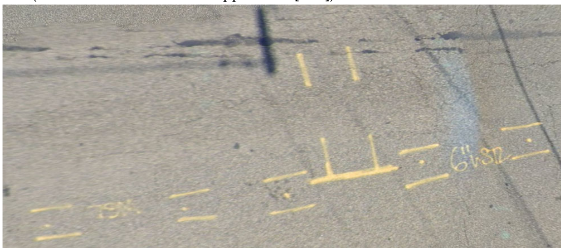
Figure 2. An example street marking we used to record suspected pipeline material and size (in this case 6" diameter, wrapped steel [STL]).
