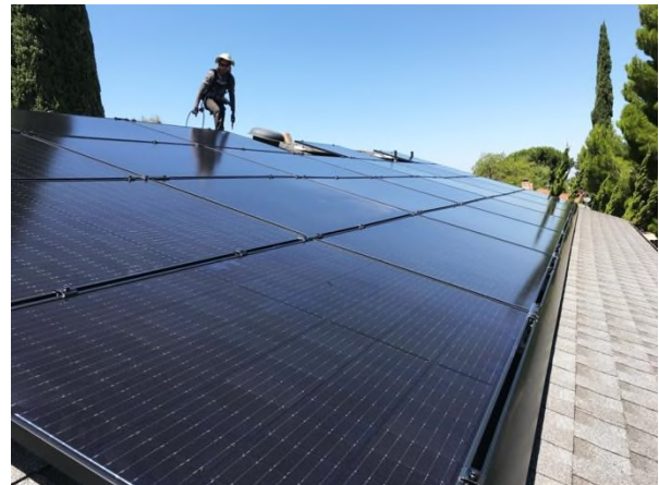
Solar panels installed by Sunrun employee
