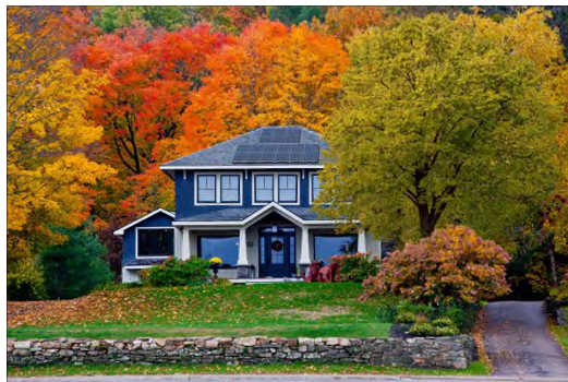
Installed solar panels in New England
