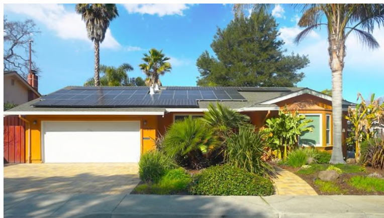
Rooftop solar installation
