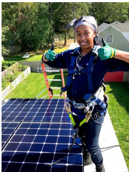
Installer with solar panels
