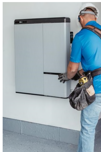
Installing a home solar battery
