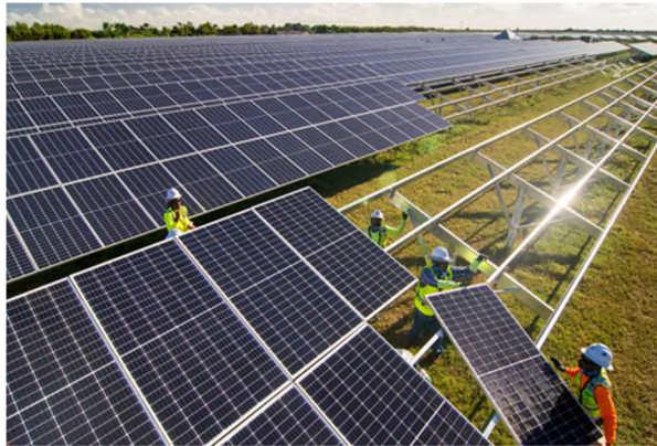
Figure 12. Solar Power Plant Under Construction
