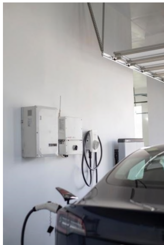
Electric vehicle charging with inverter and home solar battery
