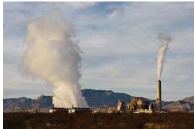
From the aquifers to the plant: Where surface water is scarce, operators of power plants such as the Apache Generating Station, a coal- and natural-gas fired plant in southeast Arizona, usually tap alternative sources of water. In parts of the Southwest and Texas, thermoelectric power plants tapped groundwater for more than half of all the water they consumed in 2008.
