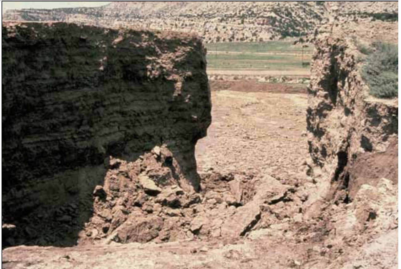
EPA Photo, Wikimedia Commons Church_Rock_uranium_mill_tailings_dam_breach.jpeg
