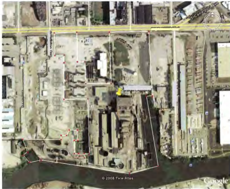
Figure 5-3: Space constrained site; Plant No. F382
