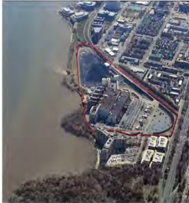
Figure 5-5: Space constrained site; Plant No. F235
