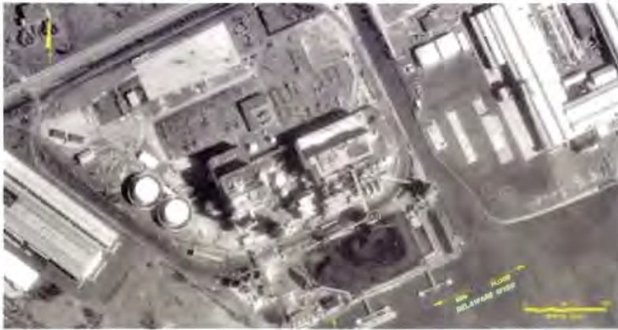
Figure 5-1: Space constrained site; Plant No. F465
