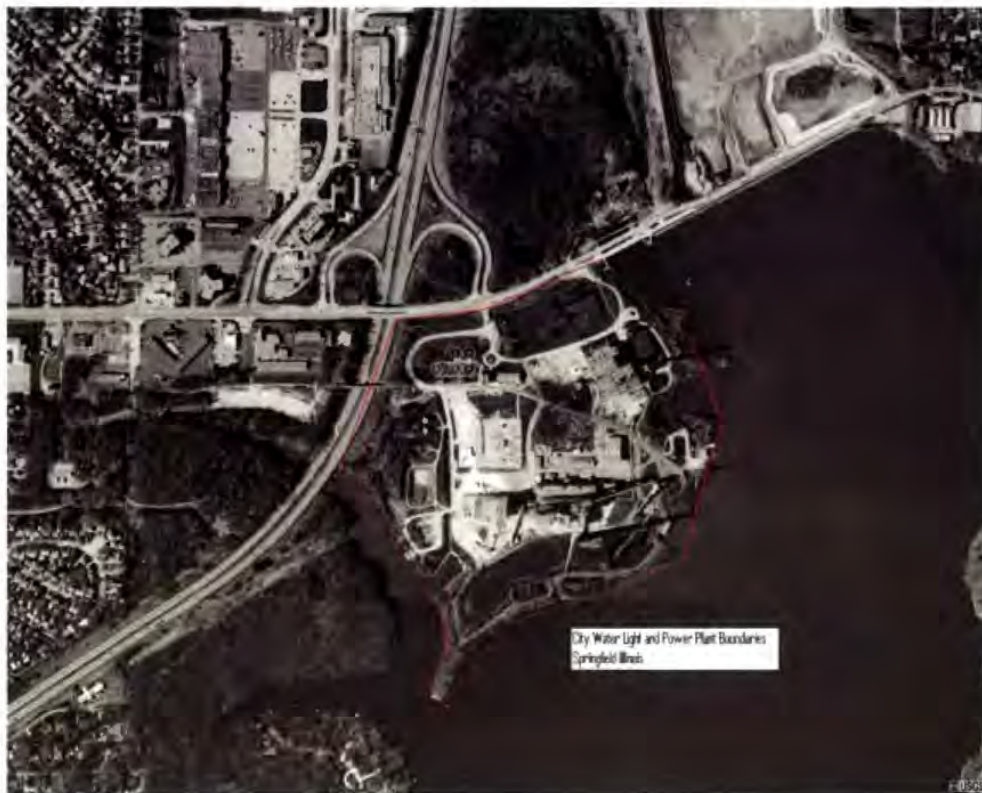
Figure 5-7: Space constrained site; Plant No. F390
