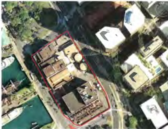
Figure 5-2: Space constrained site; Plant No. F485
