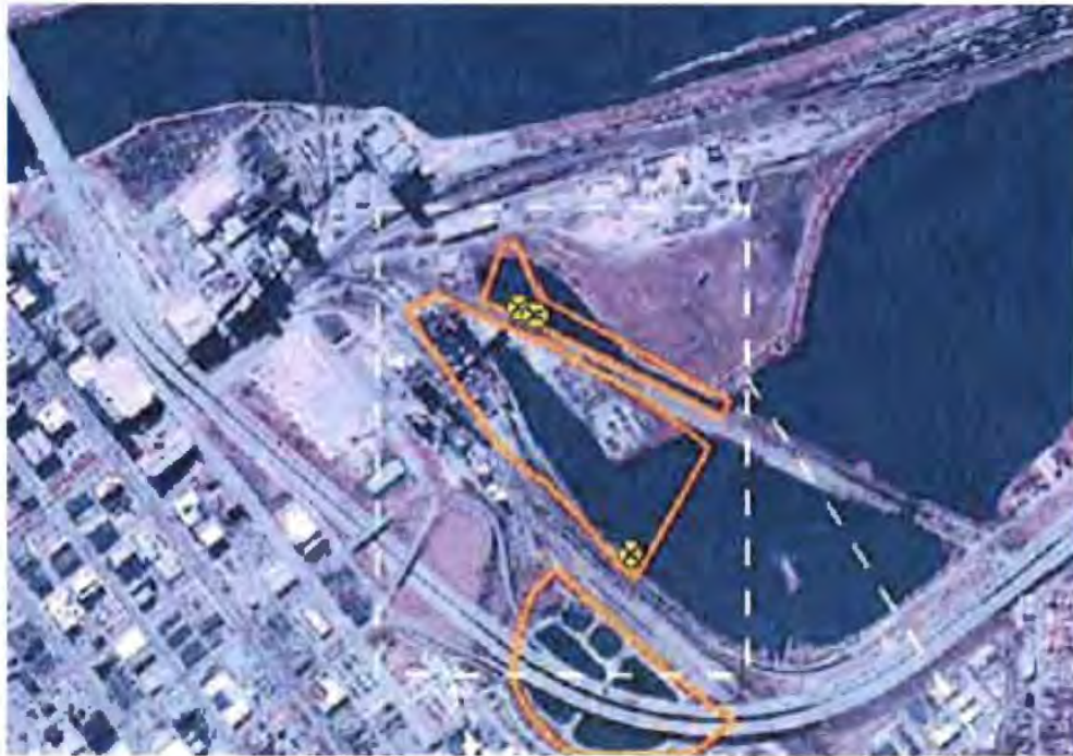
Figure 5-6: Space constrained site; Plant No. F356
