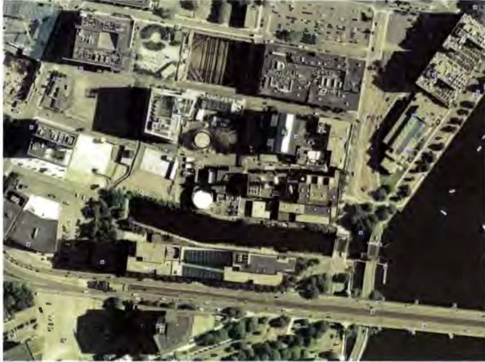
Figure 5-4: Space constrained site; Plant No. F124
