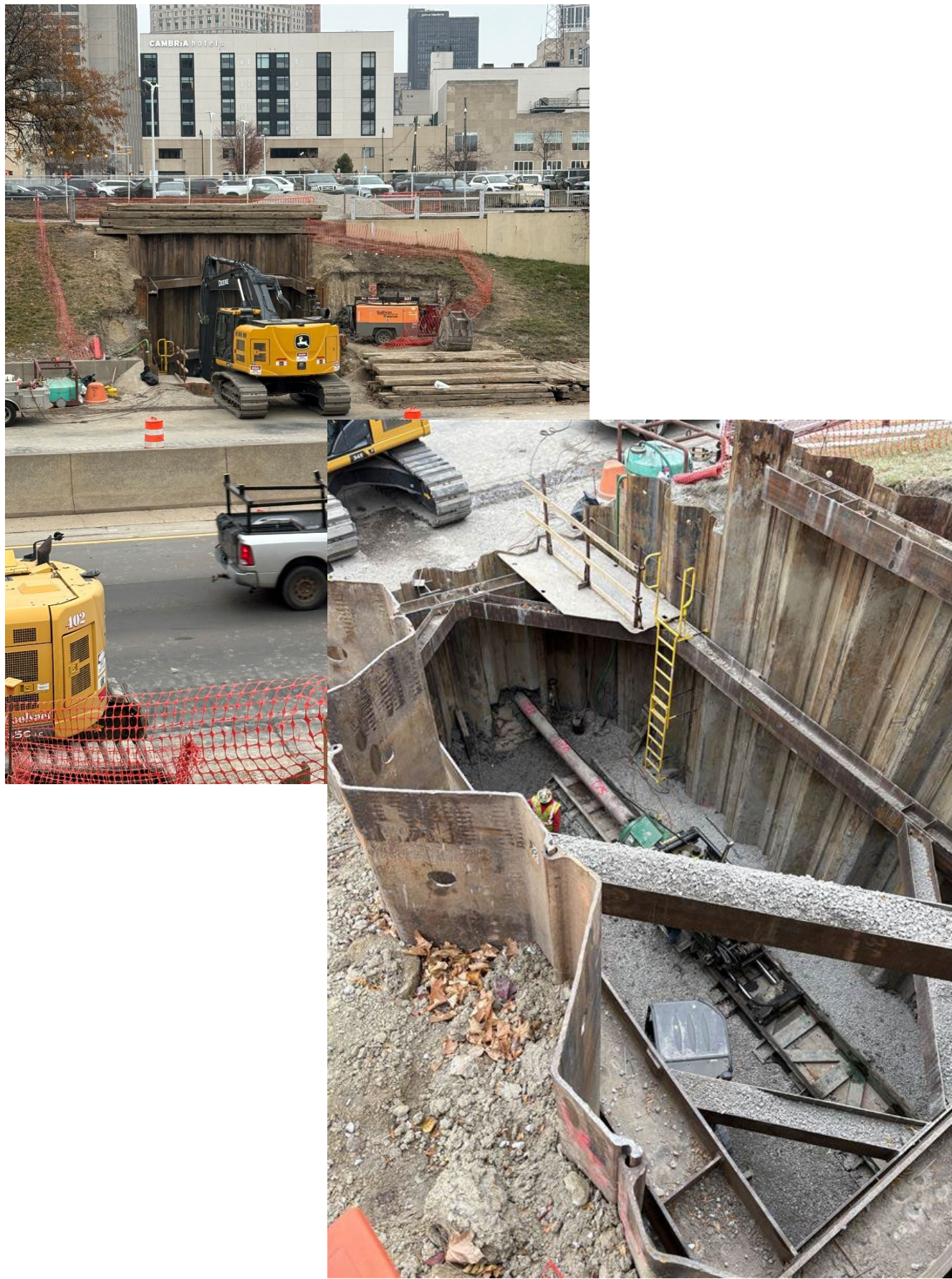
Southwest Detroit Freeway Crossing
