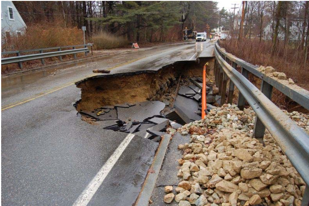
Figure 6.4 An example of unexpected severe erosion caused by flooding in Dover, New Hampshire, April 2007. 208
