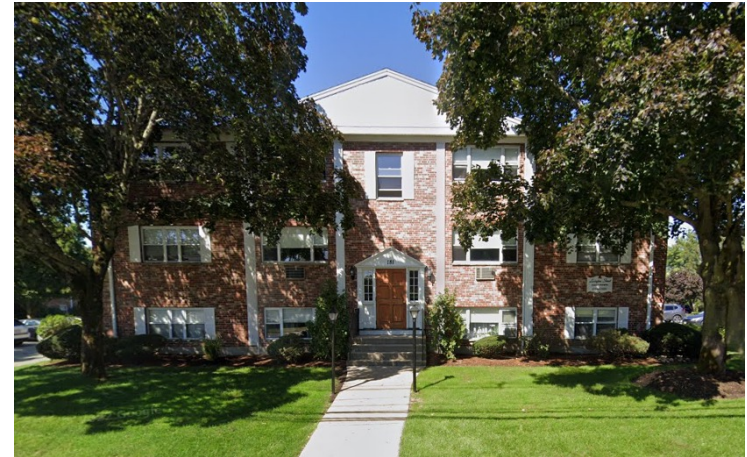
181 LEXINGTON STREET WITH BOILER ROOM
